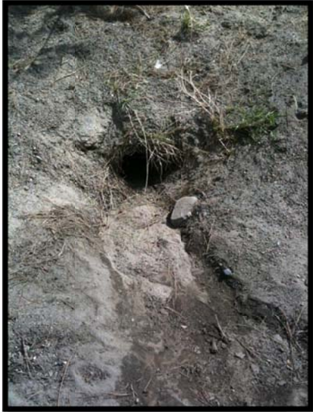
Figure 2. Inlet 2 in Bed Filter filling up with sediment. Adding a sediment can between this point and the slotted drain will help reduce further maintenance.
