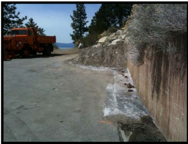
Figure 3. Drainage inlet is clogging due to runoff from stockpiled traction control material.
