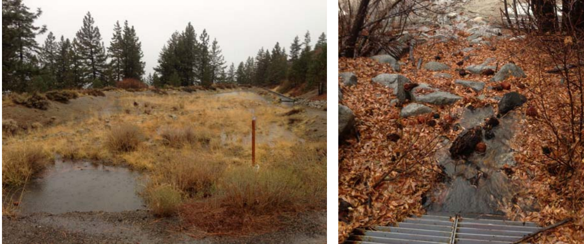
Figure 1. Left: The bed filter during the storm. Right: Outlet from bed filter to Lake Tahoe.
